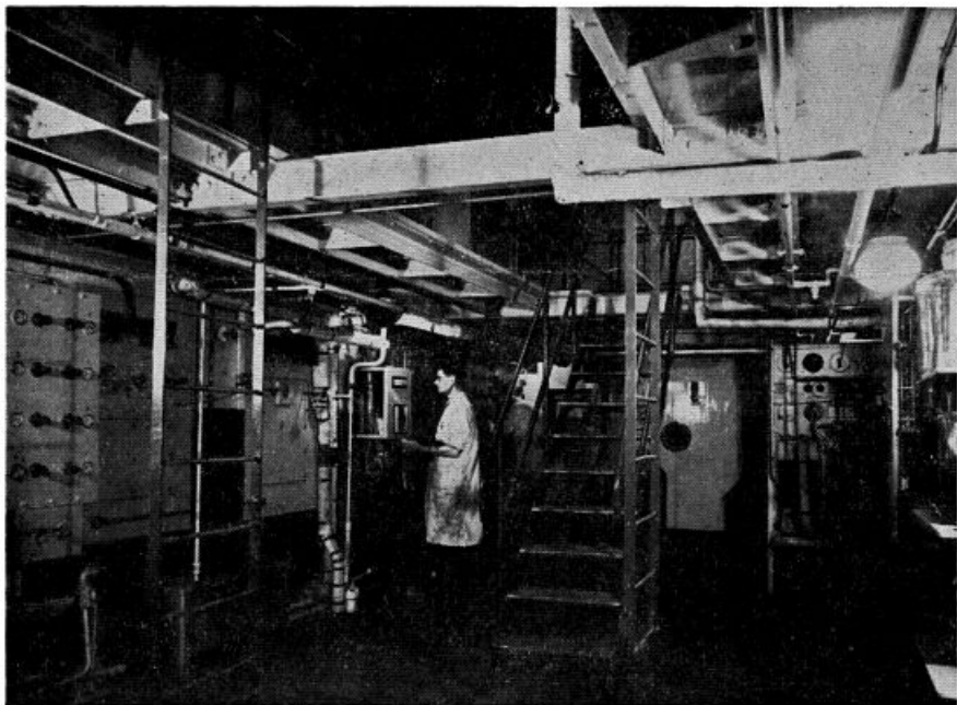
Fig. 8. The control room of the acetylene high-pressure building.
